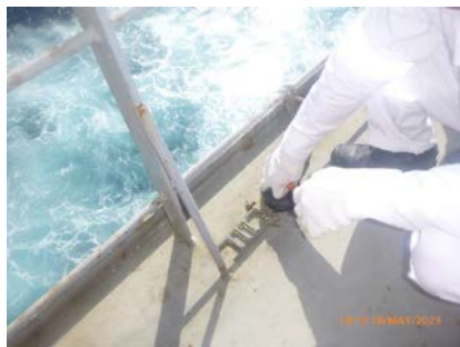
Rechecked Scupper plugs
